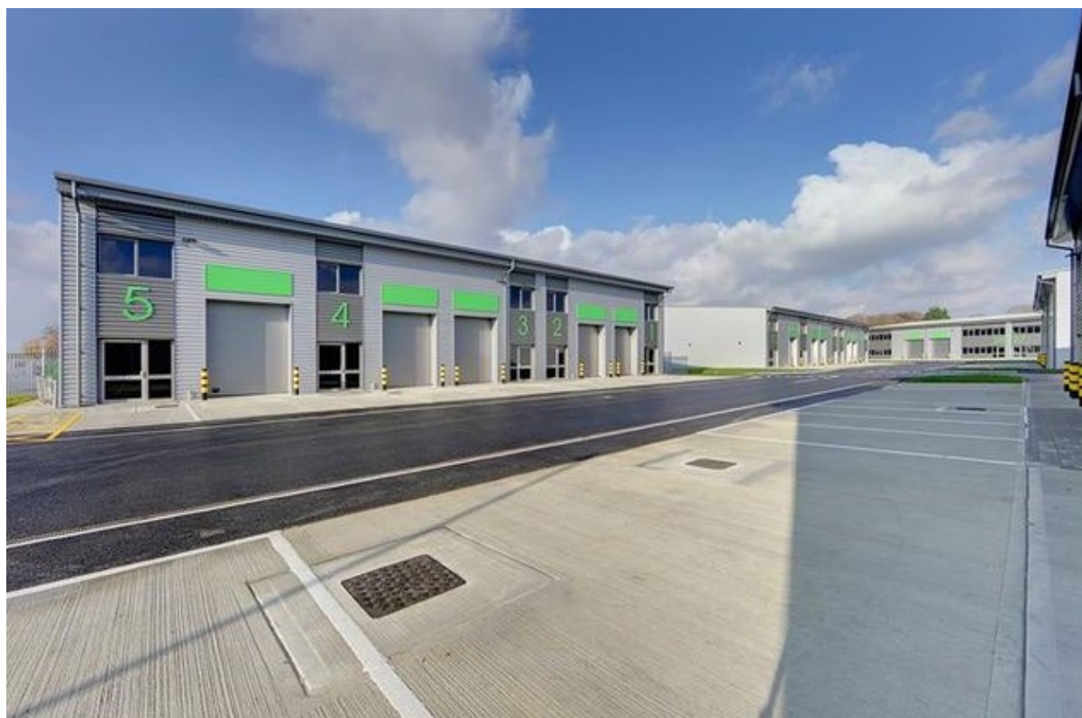
Figure 3: Plot 3 industrial units as completed.
